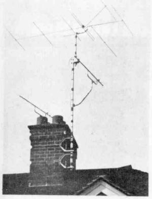
The lower mast carries a fixed TV array plus a Stolle rotator for the Arrow 7 FM beam above (R. Smith Aerials, Luton).
